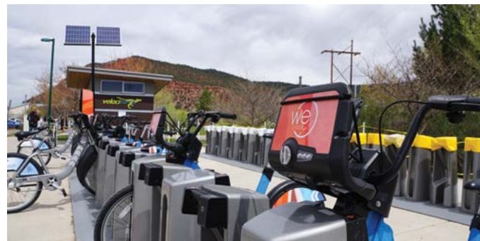
The Carbondale Park & Ride WE-cycle station nearing the end of construction in May.
