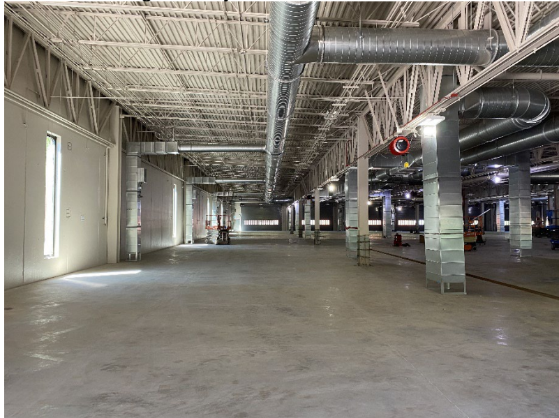
Inside the New 60 Bus Storage Facility
