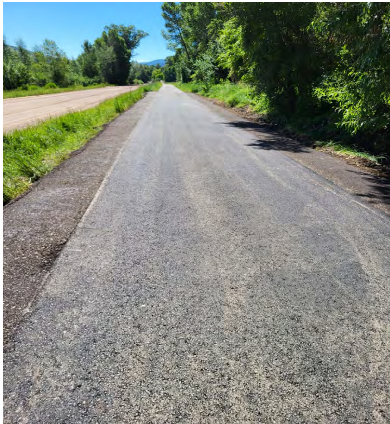
Photo – completed section of asphalt repair...smooth!
