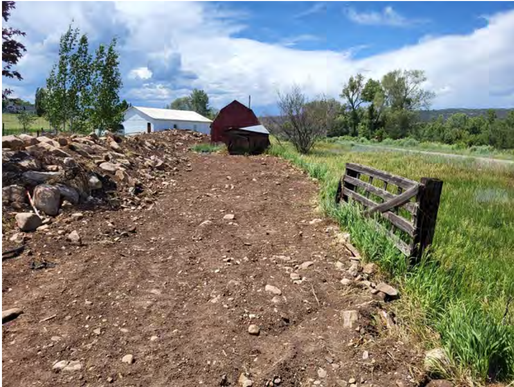
Start of the Berm Removal
