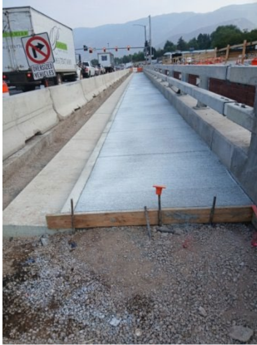
New sidewalk on northbound side of SH-82
