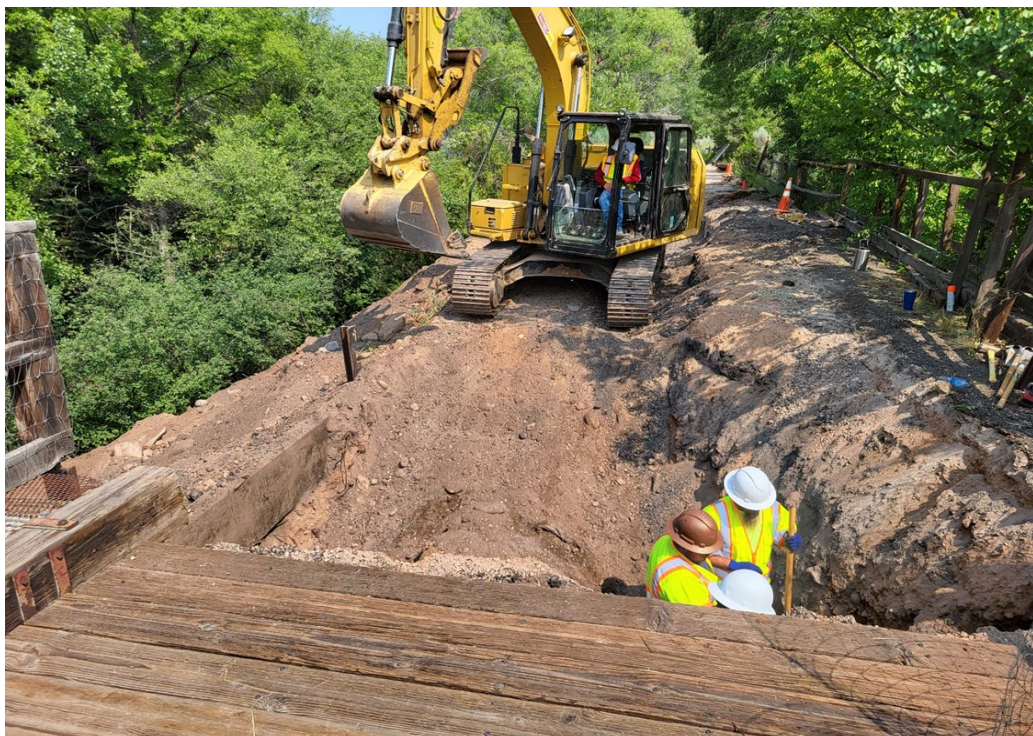
The Meridian crew is working on the Roaring Fork Bridge repairs
