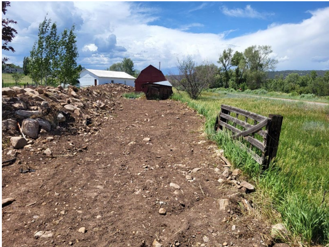
Start of the Berm Removal
