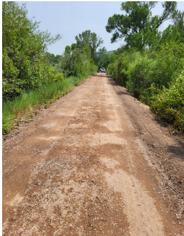
Holmes Excavation is prepping subgrade and getting ready to pave
