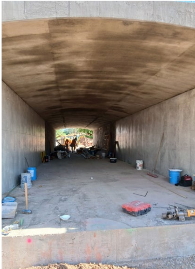
Tunnel under 27 th Street
