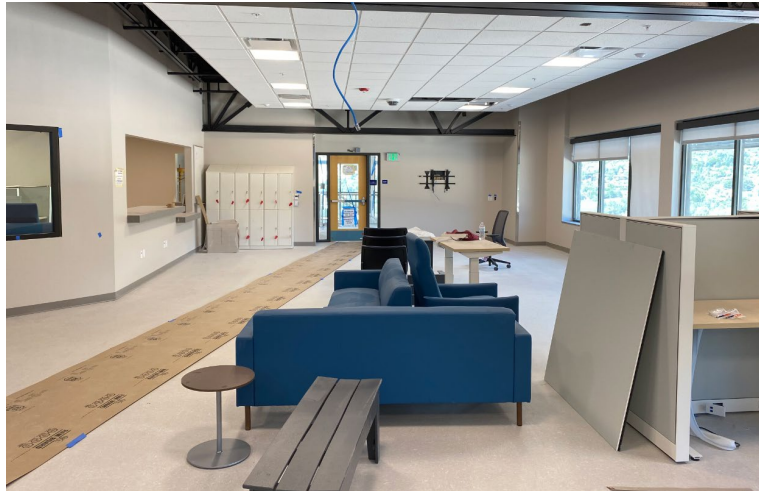
Interior of Glenwood Operations Center
