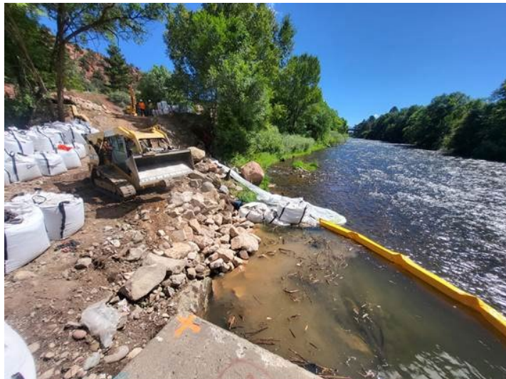
Roaring Fork Trail Bridge in Carbondale – Abutment Repair
