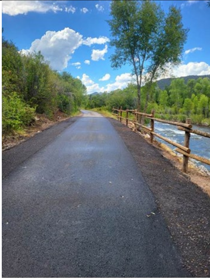
Completed Trail Section of RGT
